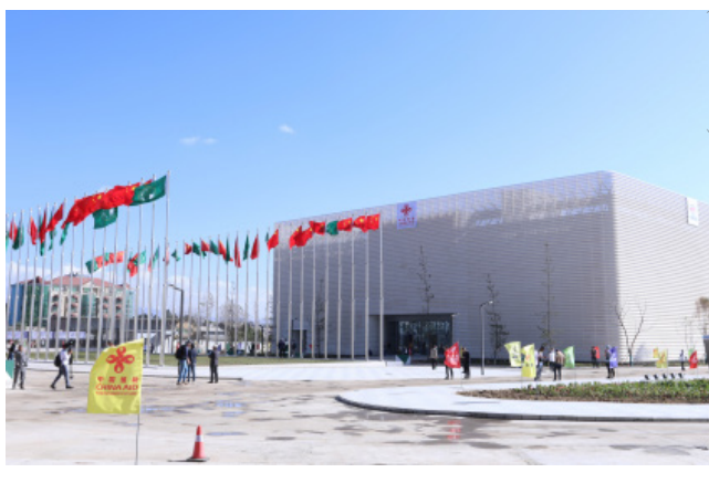
The Laboratory Building of the Africa Centers for Disease Control and Prevention headquarters project.
