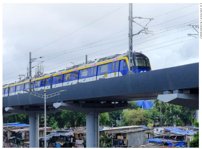
This is a part of the metro project, under loans from the New Development Bank, in north Mumbai, India, on June 22, 2023.
